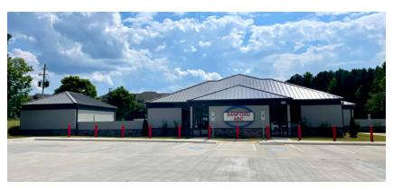
The completed building includes a newly constructed 4,435-sq ft. warehouse addition with two office areas, a break room and restrooms. An existing 2,582-sq.ft. CMU structure was completely renovated with new sheetrock walls, exterior EFIS façade and new installation of electrical, lighting, plumbing, HVAC ducts and equipment and a standing metal roof system with gutters and downspouts.
