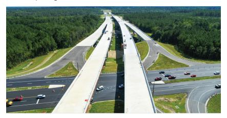
The magnitude of the bridge construction on this project was unlike any SCI had previously completed. The bridge elements were extremely large, and substructure concrete pours ranged from 40 CY to more than 400 CY. With the increased size came increased challenges (i.e. complex formwork, rigging, and larger equipment requirements). However, SCI and its team members rose to the challenge to plan, execute, and deliver this impressive section of I-295.
