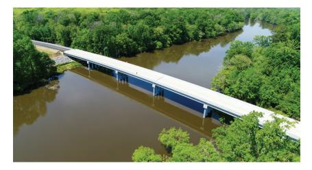
Bridge 138 and Bridge 139 in Craven County, NC, were in poor condition and nearing the end of their service life. With only a fourmonth window to accomplish "in-water" work, scheduling and material acquisitions were essential to the success of this project. Installing four temporary work bridges coupled with the installation of eight pipe pile bents for the bridge foundations proved challenging, but SCI's team members accepted the task and completed a quality project.
