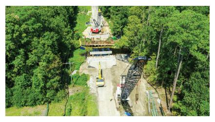
Within a tight timeframe of only six months, SCI demolished the original structure and completed the new two-span structure and approach work. SCI also paved the bridge and added markings to complete the project. To protect the environmentally sensitive areas of this project, an impervious dike and dewatering operation was required to be installed before completing each end bent.
