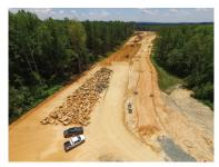
The work required developing a large number of homesites amid challenging topography and rock excavation. Sanford Contractors worked with the owner, engineer, and design team to minimize and manage the earthwork and rock manipulation, and helped develop plans and budgets for the various phases even before jobs were contracted. As a result of proactive collaboration, the percentage of change orders processed was less than 1%.
