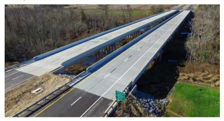
Serving as a subcontractor to Branch Civil—the project's General Contractor for NCDOT—Sanford Contractors collaborated closely to identify critical path structures. Over the course of the project, Sanford Contractors built more than 3,600 linear feet of bridge deck across seven sets of dual bridges, carefully timed to support Branch Civil's grading operations.
